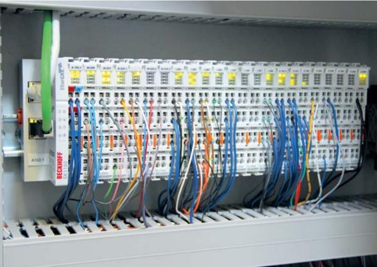
The EK1100 EtherCAT coupler integrates the numerous EtherCAT terminals into the control system, e.g. EL3202 2-channel input terminals for resistance sensors and EL5101 incremental encoder interface terminals.
