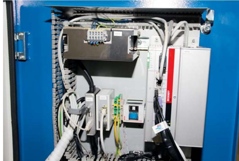
The C6920 Control Cabinet Industrial PC with its Intel® Celeron® 1.9 GHz dual-core processor offers ample computing power for demanding circular interpolation functions.
