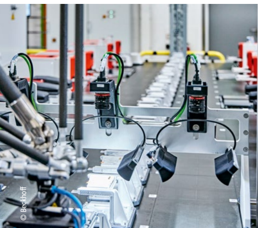
The bridge with the vision systems which is positioned over the three lanes captures the DataMatrix code of each terminal as it passes through, which is then "married" to the ID of the XPlanar mover.
